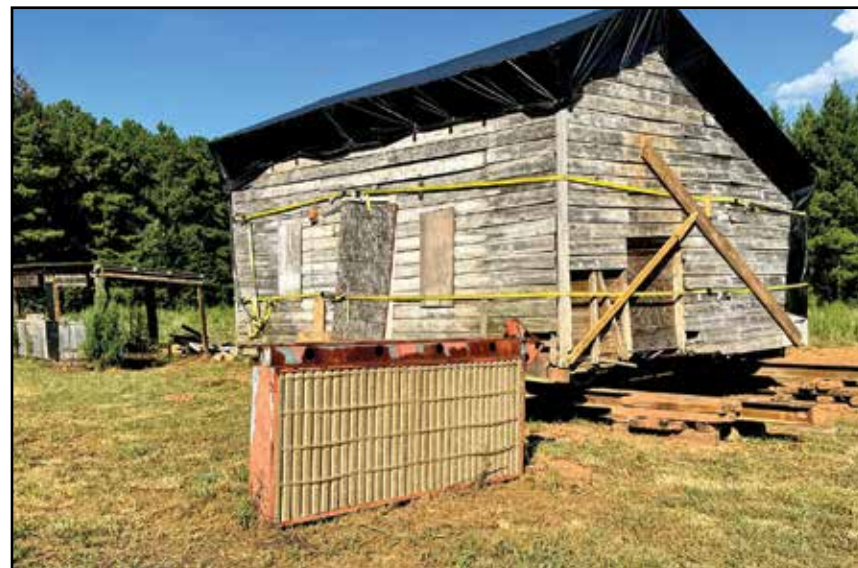
The Alexander Farms tenant house has been relocated to Blackberry Ridge Farm in Huntersville / Jason Benavides photo
