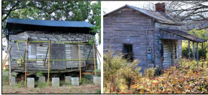
Tenant house in 2026 (left) and 2022 (right) / Cornelius Today photos
