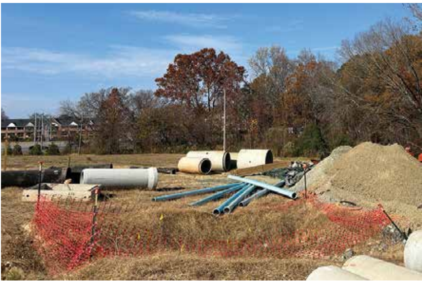
Novant is proposing an 11,400-square-foot freestanding emergency room roughly two miles north of the new Atrium emergency room.
