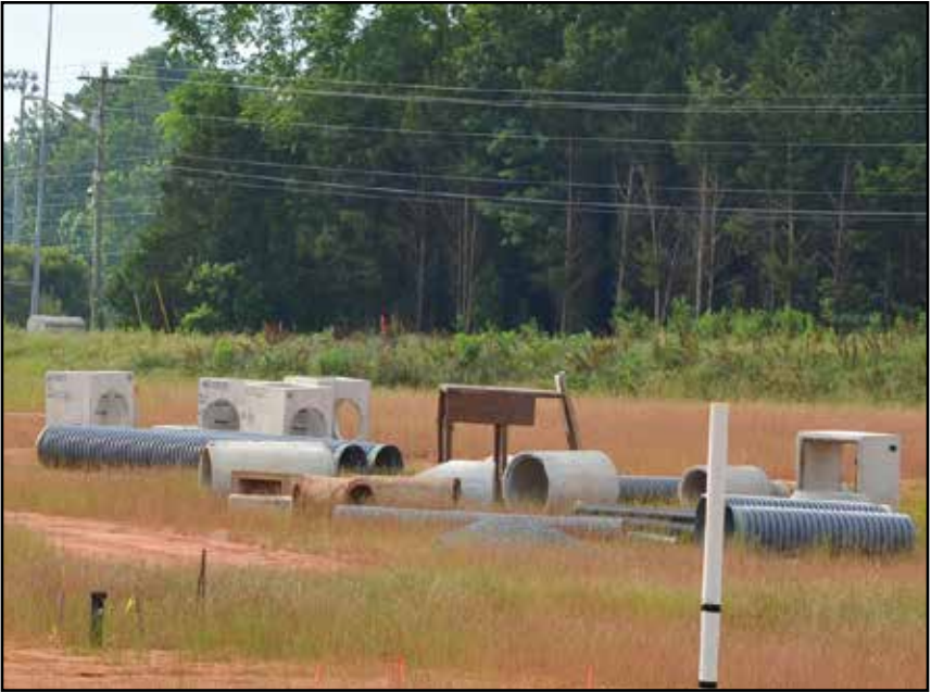
Construction at Alexander Farms / File photo by Jason Benavides
